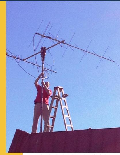
**Above**: Peter Landon, KE6JPM, on the roof at Soleado Elementary School adjusting the antenna rotation system for tracking satellites and the International Space Station using NOVA software.
