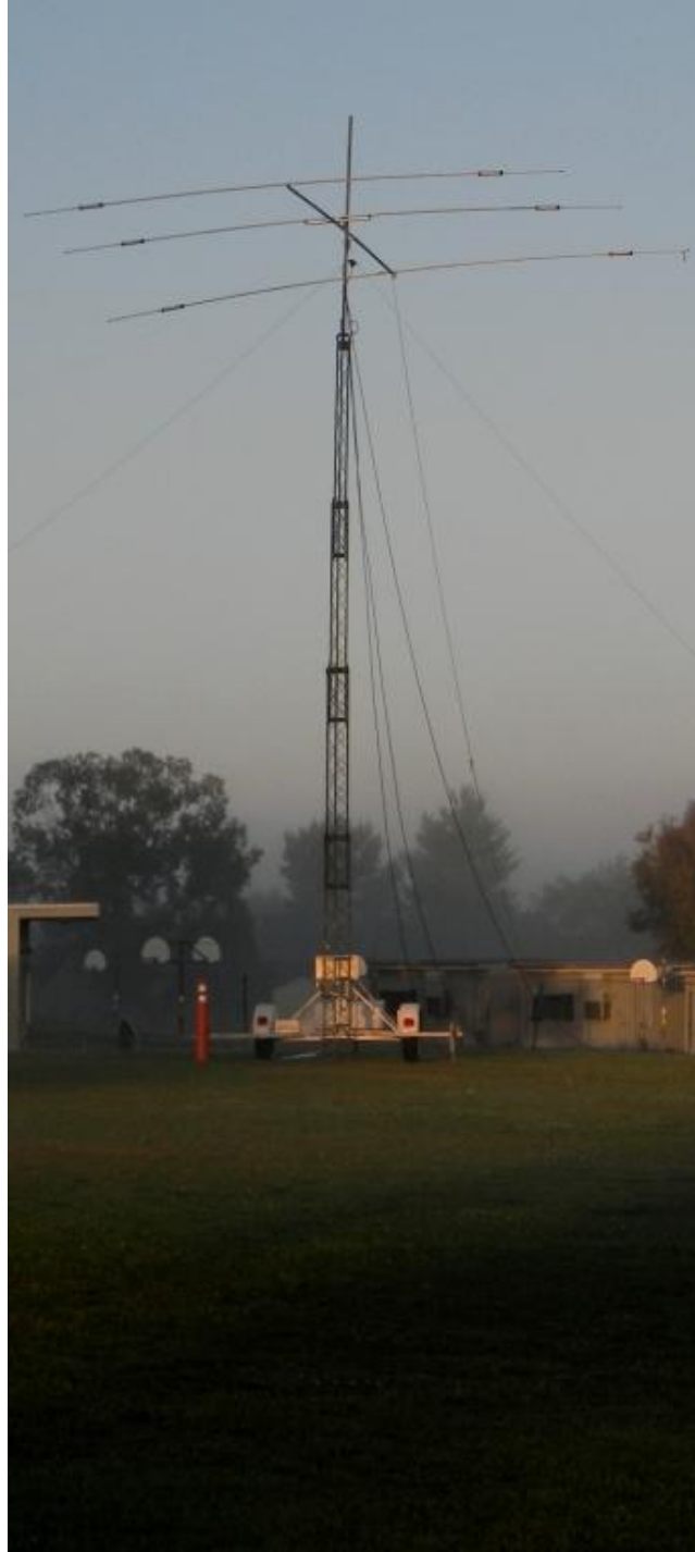
The PVARC’s tower trailer at sunrise on Field Day.
