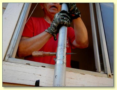
**Ham radio ingenuity:** After a locking pin does not pop out to hold a mast section, Ray, N6HE, applies a clever solution to both support our 5-band hexbeam antenna and rotate it from inside the radio room. PHOTO: DIANA FEINBERG, AI6DF
