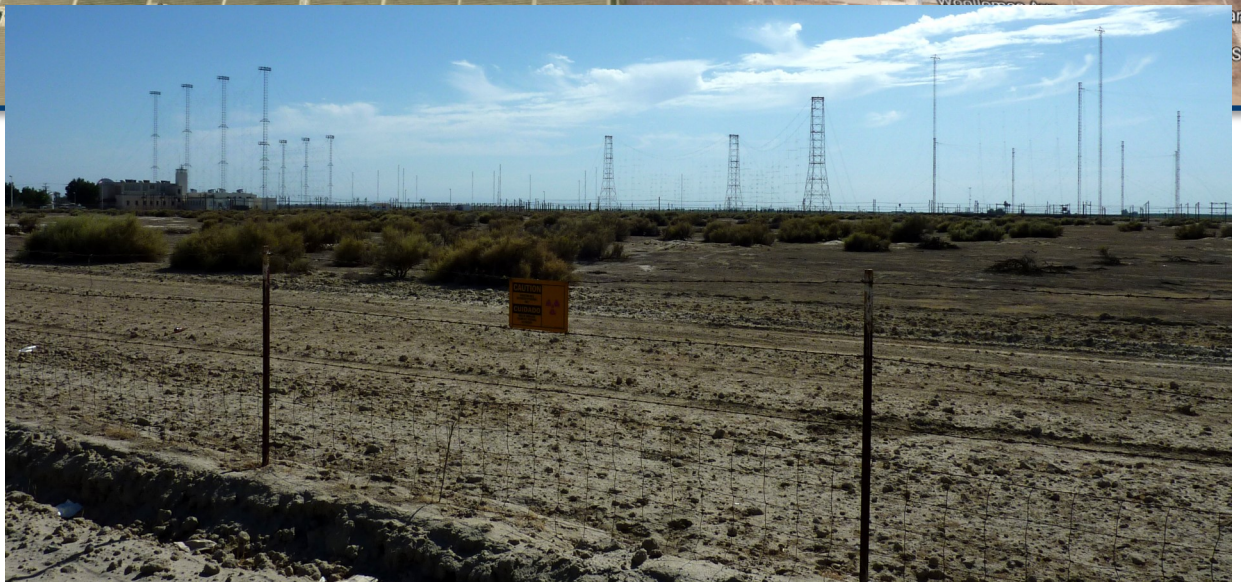
Right: The massive curtain antenna formerly used at VOA-Delano. PHOTO CREDIT: BOBAK HA'ERI (OWN WORK) [CC BY 3.0 (HTTP://CREATIVECOMMONS.ORG/LICENSES/BY/3.0)], VIA WIKIMEDIA COMMONS
