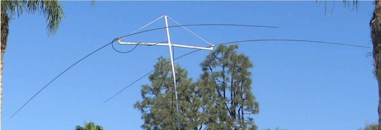
Figure 2. 17m 2-element antenna erected for testing at approximately 20 feet above the ground; this Yagi configuration uses two MFJ-2299 dipole antennas (one modified as described in the text) supported on a boom made of PVC pipe, with the two elements spaced 10 feet apart, or approximately 0.18\lambda element separation [Note: \lambda (wavelength) at 18.1MHz = \sim 16.6 m or \sim 54.4 feet; therefore, 10' = 0.18\lambda ; element spacing from 0.15\lambda to 0.25\lambda is considered acceptable, with little variation in antenna gain.] Boom sag was countered by use of support cords attached to each end of the boom. The slight sag of the two elements does not significantly degrade antenna performance.
