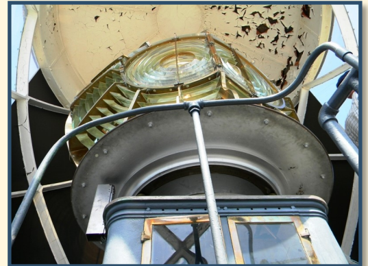
Above: The Fresnel lens—massive brass clamshell frames studded with prisms—atop Pt. Vicente Lighthouse is nearly seven feet tall including its motor base. This picture was taken August 21, 2011, during the PVARC's 2011 International Lighthouse & Lightship Weekend. After the 2012 ILLW the lens room (and later the entire lighthouse) went off-limits to visitors due to Coast Guard safety and environmental concerns. PHOTO: DIANA FEINBERG, AI6DF
