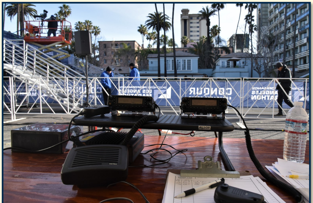
Top: View of Finish Line bridge under construction during overnight hours as seen from L.A. Marathon net control. Net Control operators were on-scene by 2:00 am.
